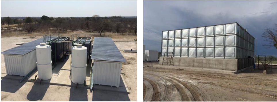
Figure 3: Existing water treatment plant and clean water reservoir (LCE, 2022)
