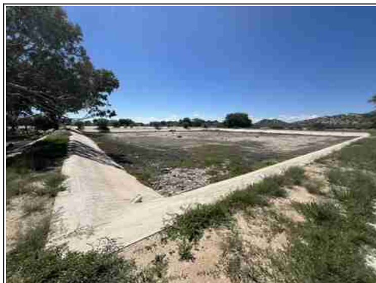
Figure 2: Some of the existing sewage infrastructure to be upgraded and rehabilitated.
