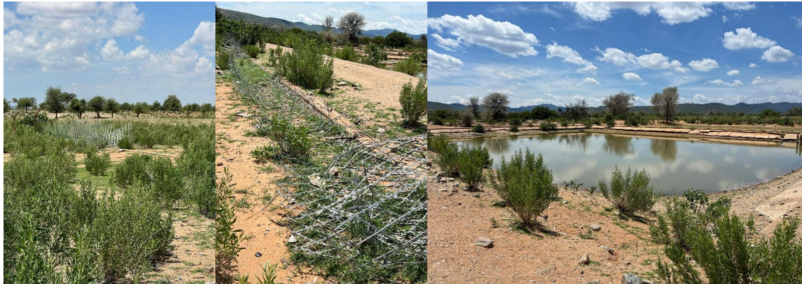
Figure 7-2: The oxidation ponds with a fallen razor diamond wire fencing and some ponds without fencing
