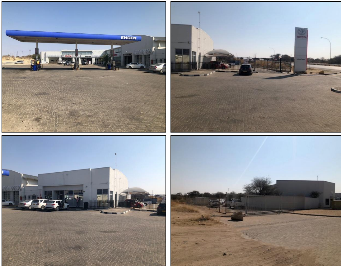
Figure 4: Main buildings on site
