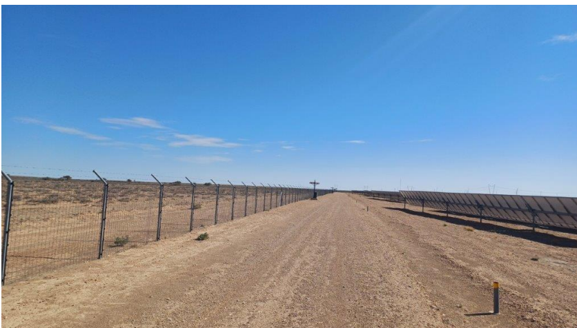
Photo 20 – View of site fence, well maintained and intact.
