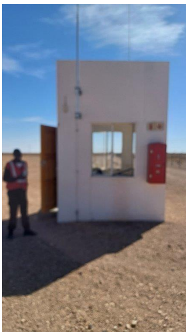
Photo 3 – View of security guard house with fire extinguisher.
