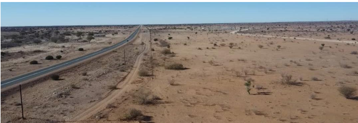
Figure 4: Shows the B1 (Trans-Oranje Highway) on the left and proposed site extending towards the right
