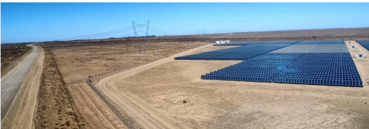
Figure 4: Shows the C17 as the main access road on the left and an illustrative layout of the on site access tracks
