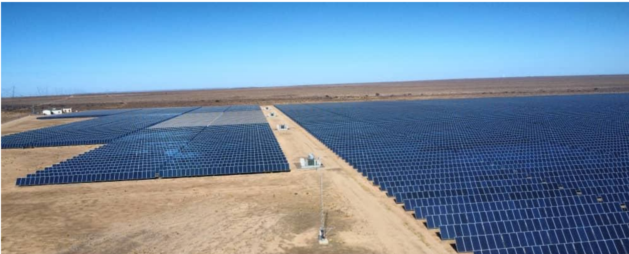
Figure 2: Illustrate the typical installation of solar panel field, similar to which Khomsec envisage to install
