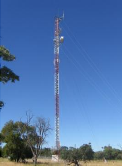
Figure 2: Typical Guyed lattice telecommunication tower structure (for visual purposes only) with guyed anchors for stability.
