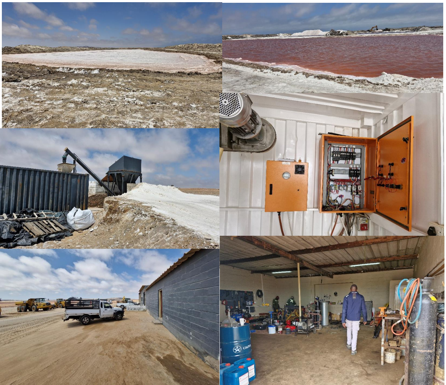
Figure 2: Overview of site infrastructure
