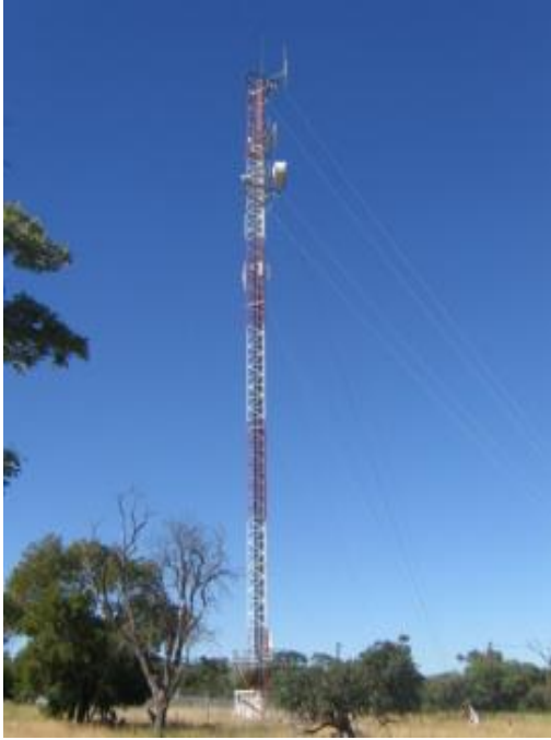
Figure 3: Typical telecommunication towers structure and form (visual purposes only)
