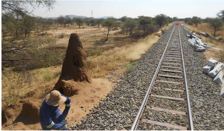
Figure 3. A termite hill that is located too close to the railway line
