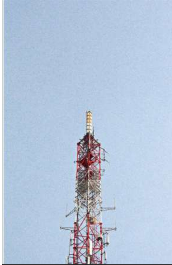
Figure 2: Typical example of a freestanding lattice telecommunication tower structure
