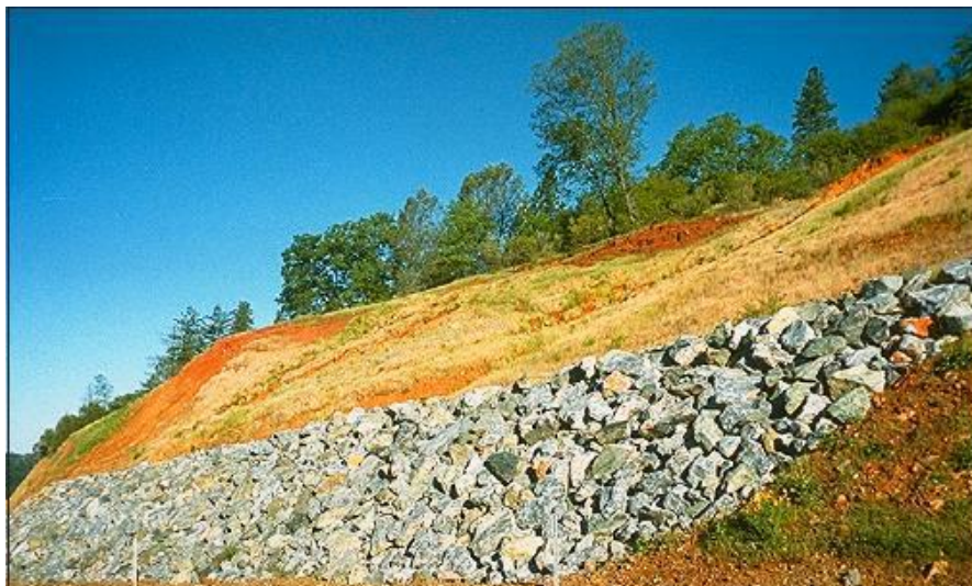
Figure 2-3: Rock buttress illustration
