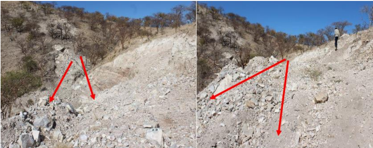
Figure 3: Evidence of trenching on targeted sites
