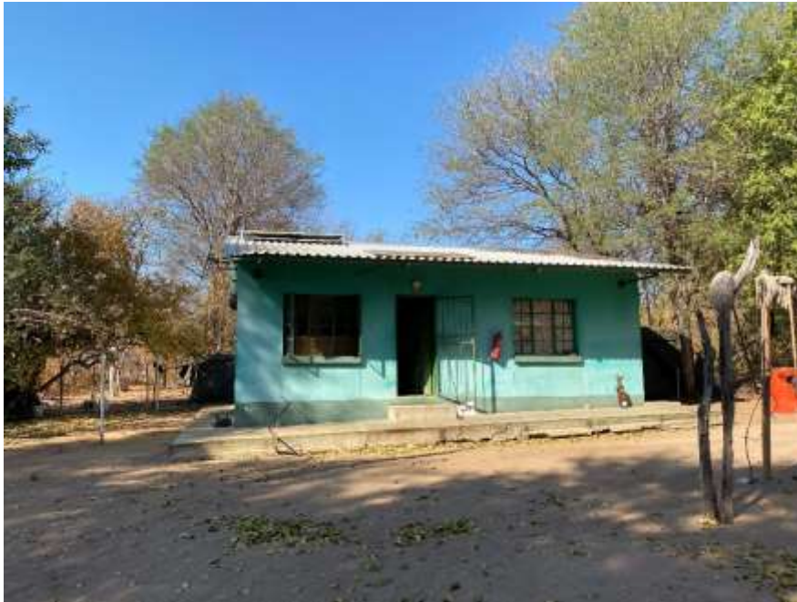
Figure 5: Current structures used by the Namibian Police and WPS staff close to the Kwando River at Susuwe.
