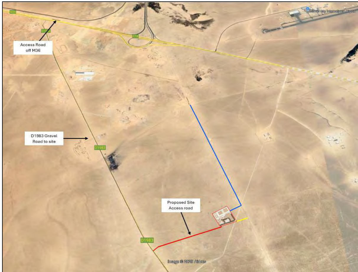
Figure 10: Site Access Road
