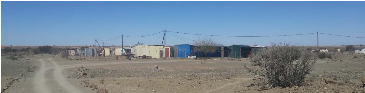
Photo 5.4.3 – View of Electricity grid in the townships
